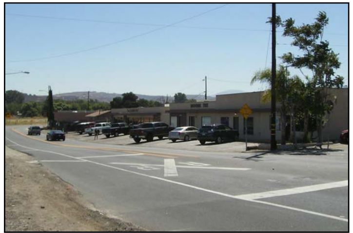
View 9: From the north side of 13th Street looking southeast.
