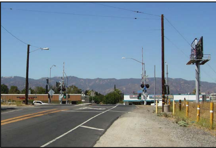
View 3: From 13th Street looking west towards the Project Site.
