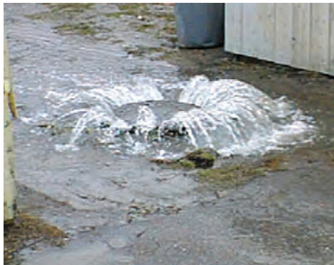
Sewer system overflow
