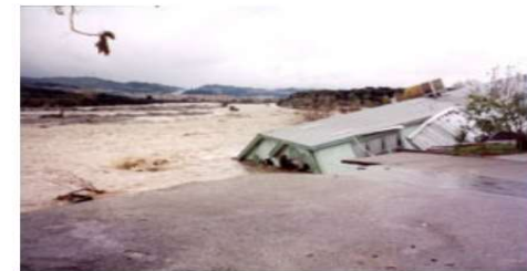
Sand Canyon Mobile Home Park 2005 Flood Damage
