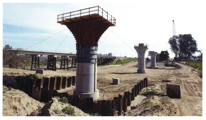
The supports for a 1,600-foot-viaduct to carry high-speed rail trains across the Fresno River are seen under construction near Madera, Calif. (Rich Pedroncelli / AP)
