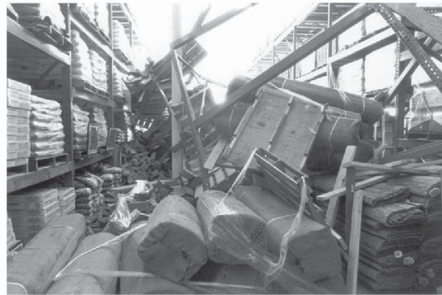
Figure 2-1 Cross-aisle collapse in the building materials section of the Santa Clarita store.
