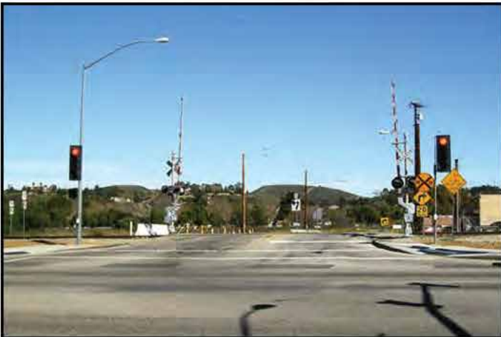
View 5: From the west side of Railroad Avenue looking east.
