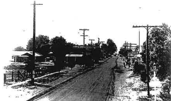
Spruce Street - 1916 (Main Street)
