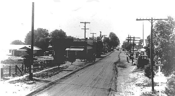
Spruce Street – 1916 (Main Street)
