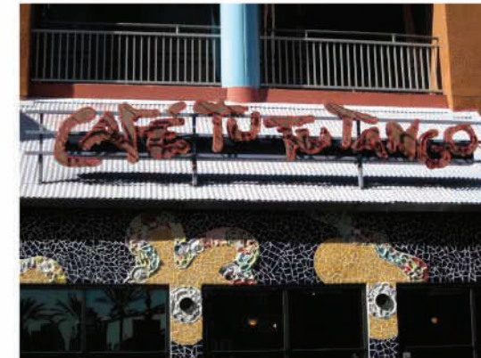
This type of sign will not be acceptable due to the exposed neon on the face of the letters (exposed neon is not allowed at Bridgeport Marketplace)
