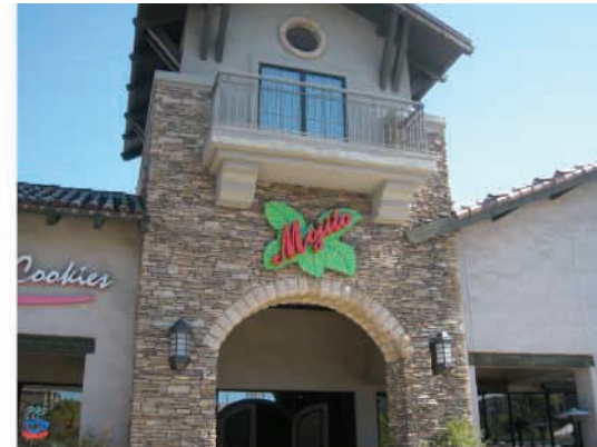
This is a great example of a creative background that also works as a wireway.
