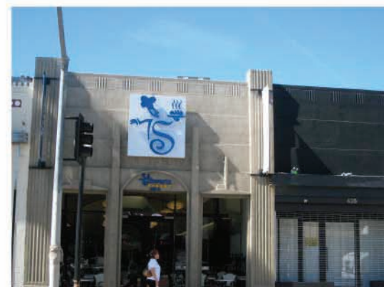
Fabricated panel with reverse channel logo pin mounted off of face, logo pieces halo illuminate at night.
