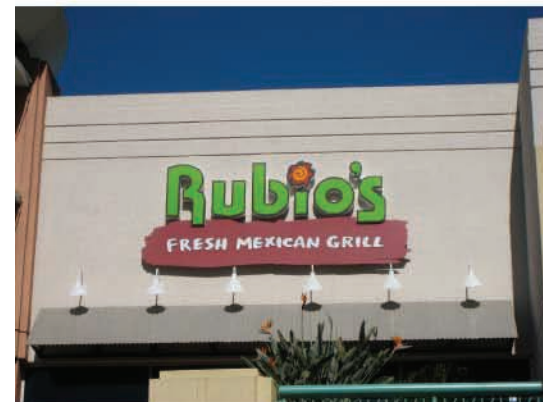
Good example of an acceptable raceway type sign, letters mount to building face but all wiring is routed thru lower cabinet with push thru copy.
