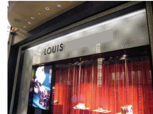
Example of letters mounted to storefront glass, this can be very effective with an illuminated soffit, letters can also be mounted to the soffit behind the glass.
