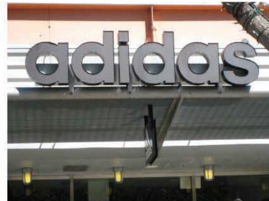
This is another example of a sign that would not be acceptable because you can see the raceway behind the letters.
