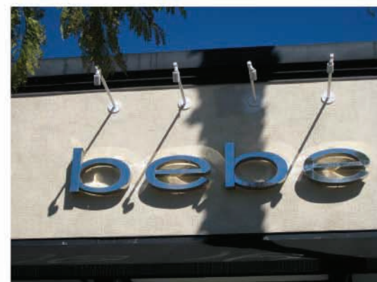
Fabricated stainless steel letters with pendant lighting.
