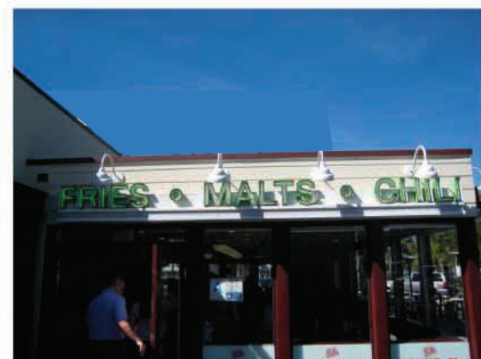
This type of sign would not be acceptable due to the raceway and the exposed neon.
