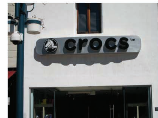
Fabricated panel with reverse channel logo / letters pin mounted off of face, logo / letters halo illuminate at night.
