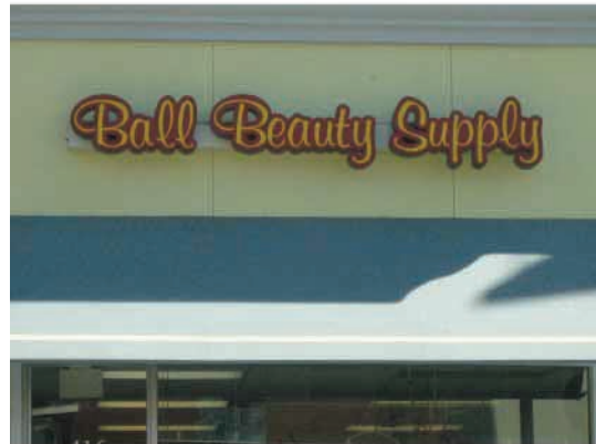
This type of sign with a visible raceway will not be acceptable.
