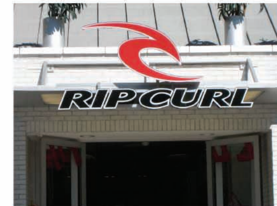
Example of storefront signage attached to a canopy, please note the raceway is not visible
