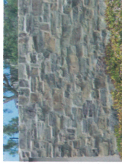
EXAMPLE OF CYPRESS RIDGE ORCHARD STONE TO MATCH OTHER WALLS AT SUMMIT OAKS
