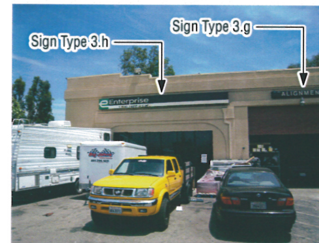
LEFT SIDE OF BUILDING #3 (WEST ELEVATION)
