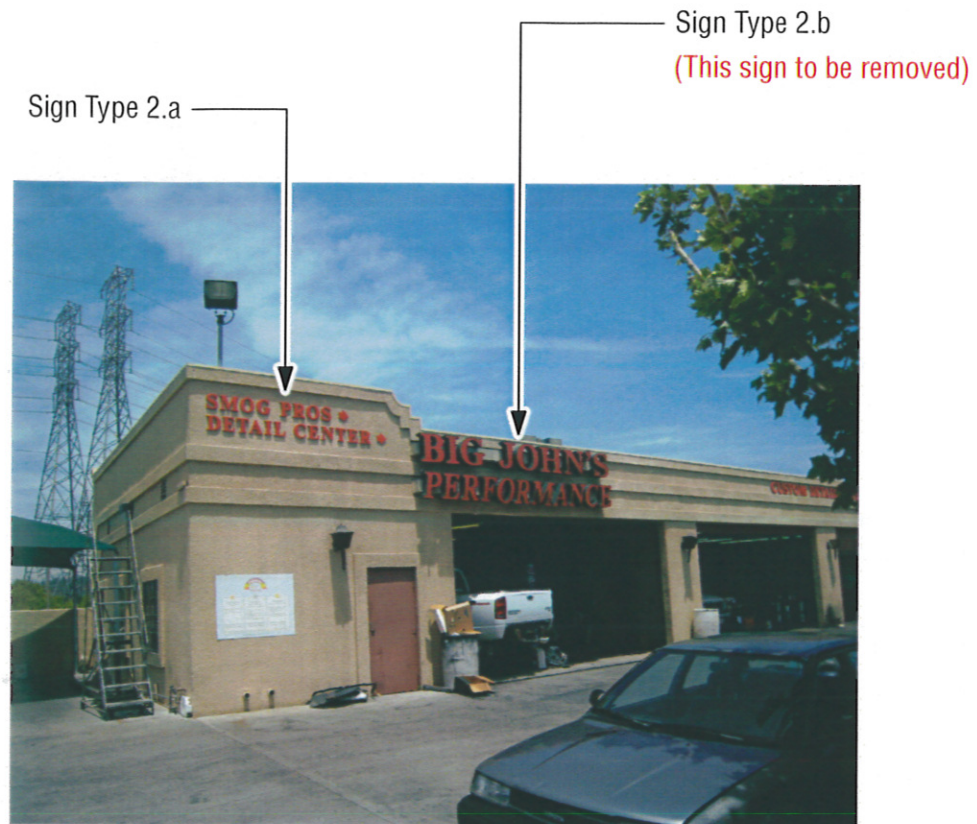
LEFT SIDE OF BUILDING #2 (SOUTH ELEVATION)
