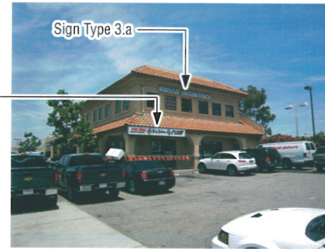
FRONT CORNER OF BUILDING #3 (SOUTH ELEVATION)
