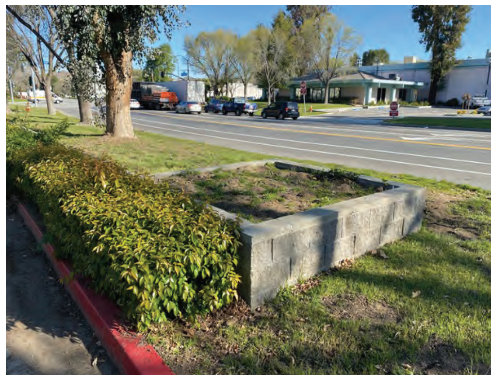
PREVIOUS MONUMENT SIGN LOCATION AT DRIVEWAY OFF OF AVENUE STANFORD
