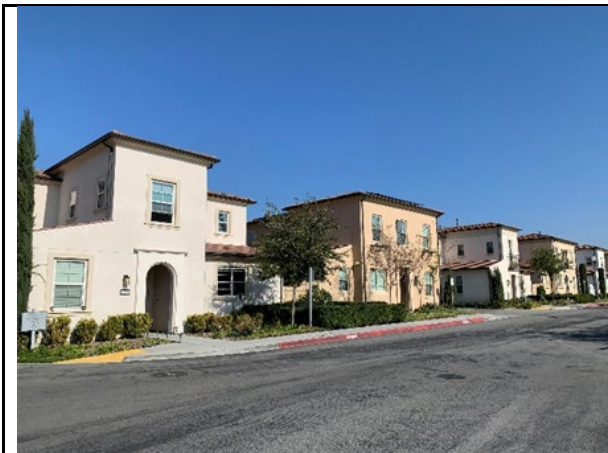
Existing: Looking Northeast
