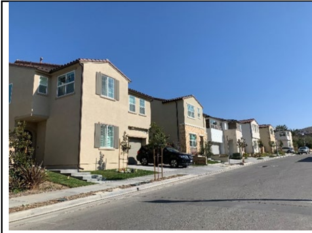
Existing: Looking Northeast
