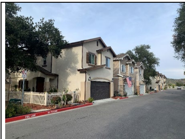
Existing: Looking Northeast
