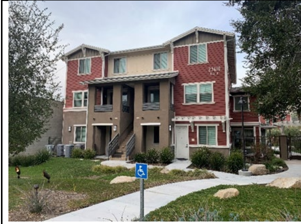
Existing: Looking North
