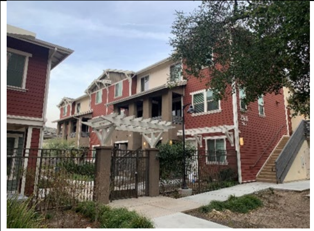
Existing: Looking Northeast
