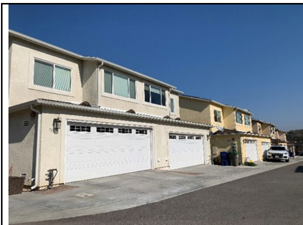
Existing: Looking Northeast
