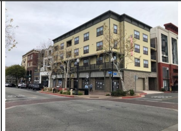
Existing: Looking Northeast
