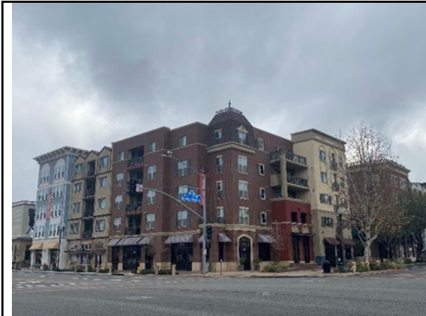
Existing: Looking Southeast
