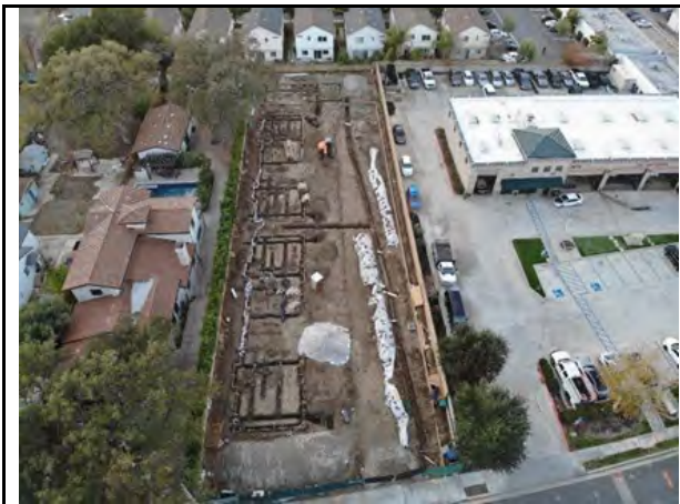
Existing: Looking West
