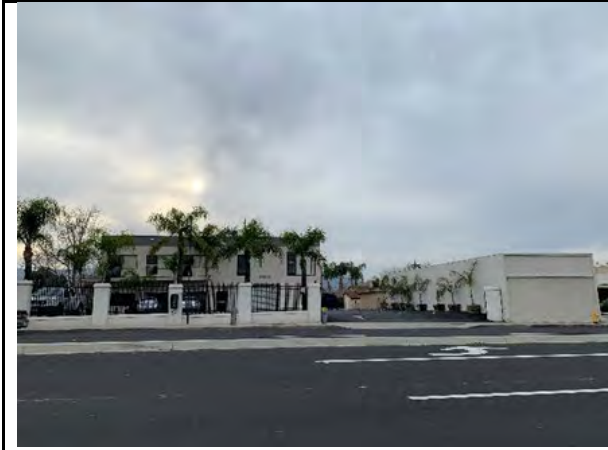
Existing: Looking West
