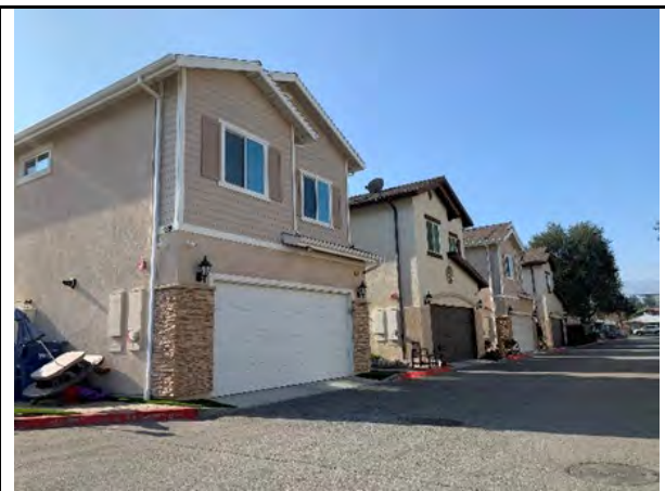
Existing: Looking Southwest
