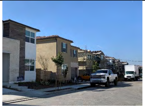
Existing: Looking Southwest
