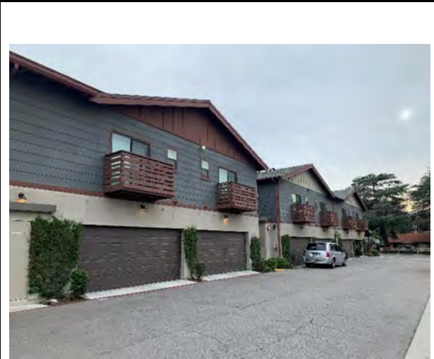
Existing: Looking Southwest
