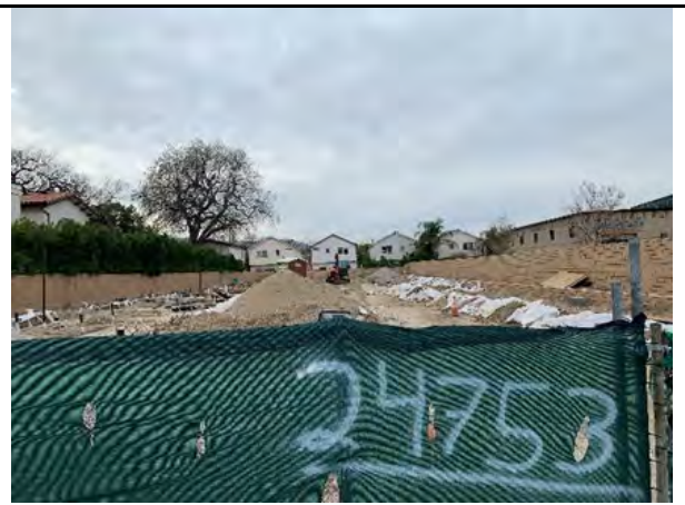
Existing: Looking West
