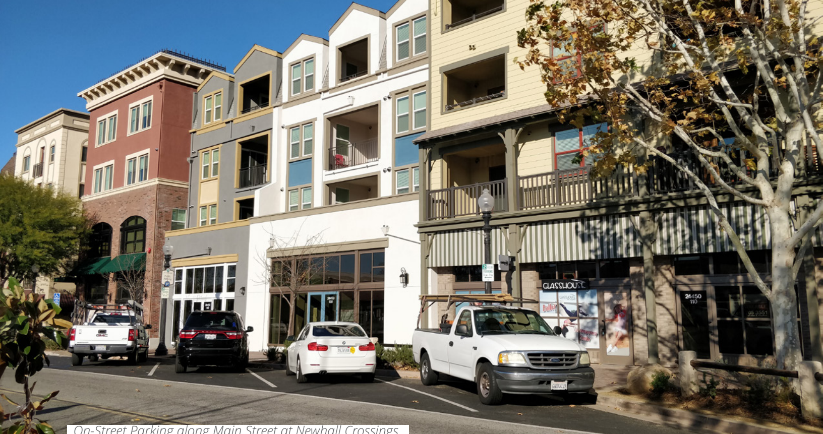
On-Street Parking along Main Street at Newhall Crossings
