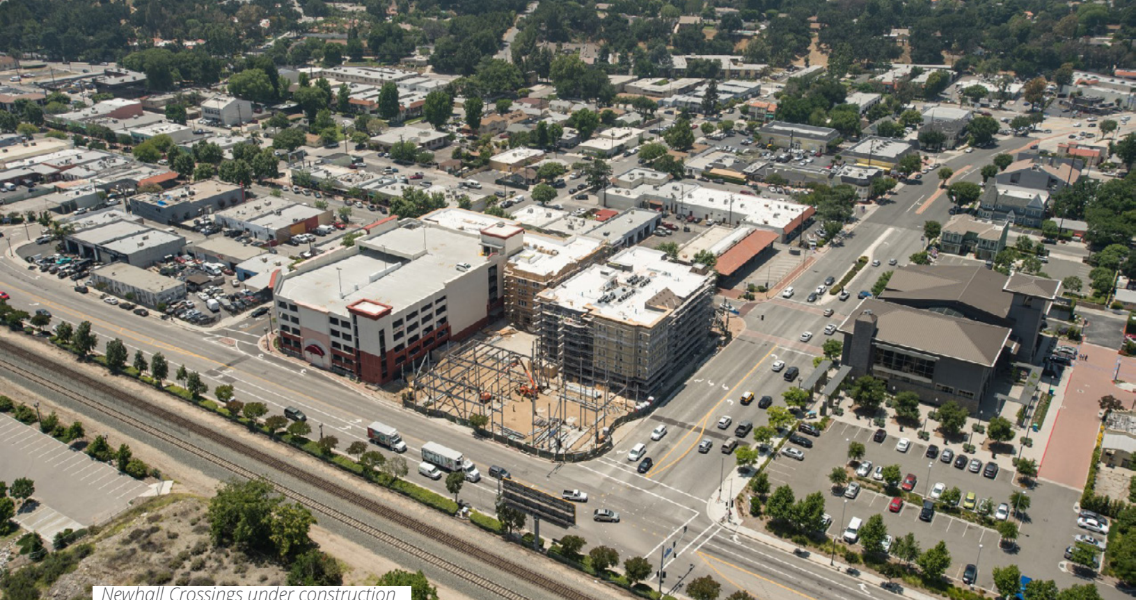
Newhall Crossings under construction
