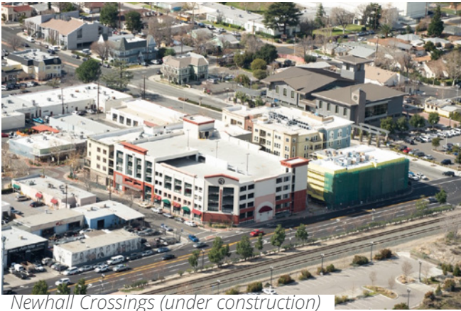
Newhall Crossings (under construction)
