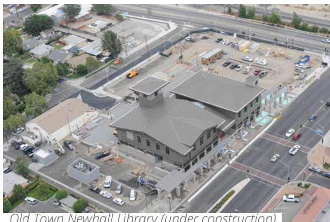
Old Town Newhall Library (under construction)
