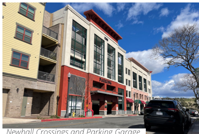
Newhall Crossings and Parking Garage
