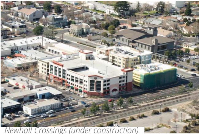
Newhall Crossings (under construction)
