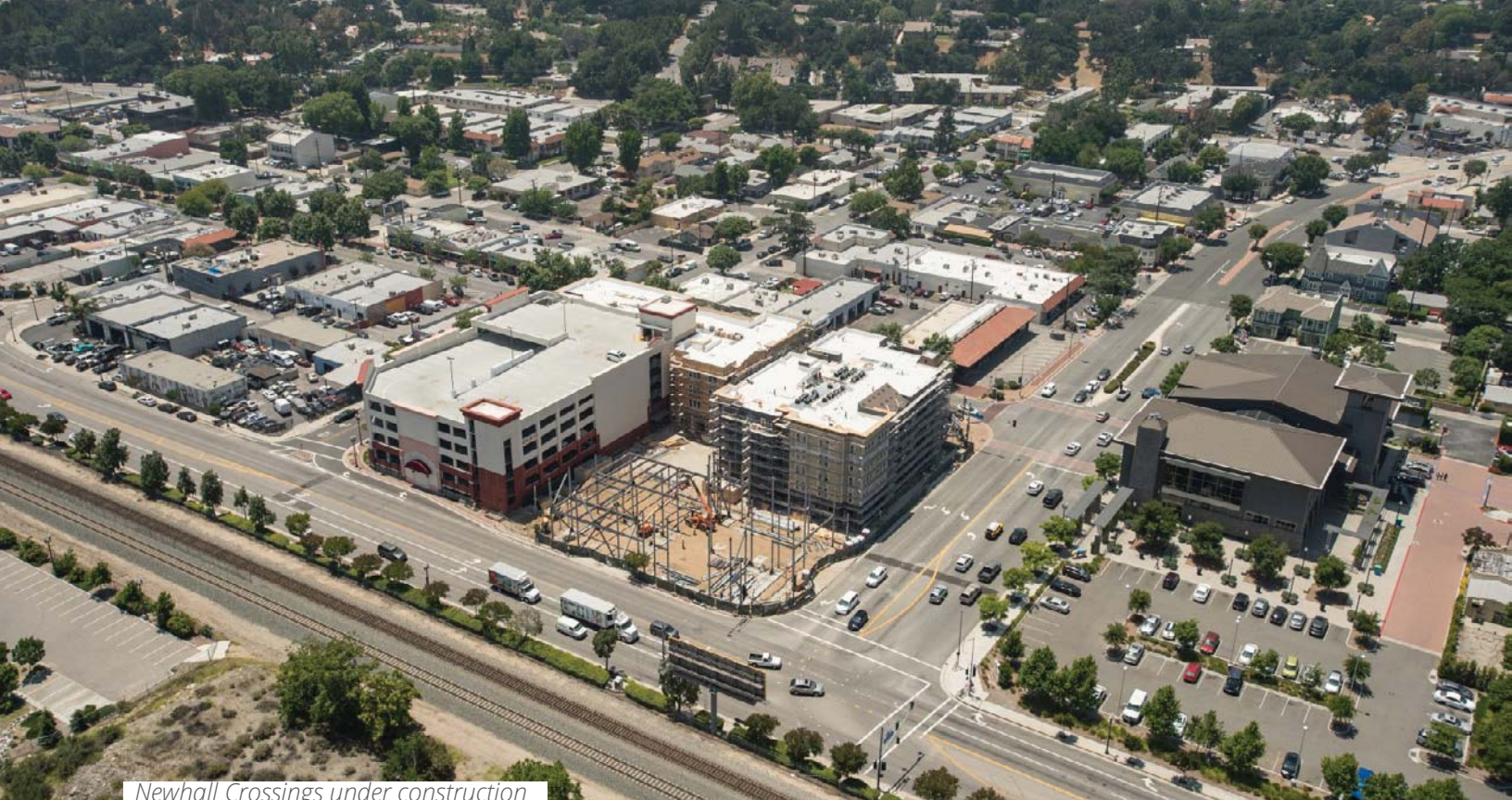
Newhall Crossings under construction
