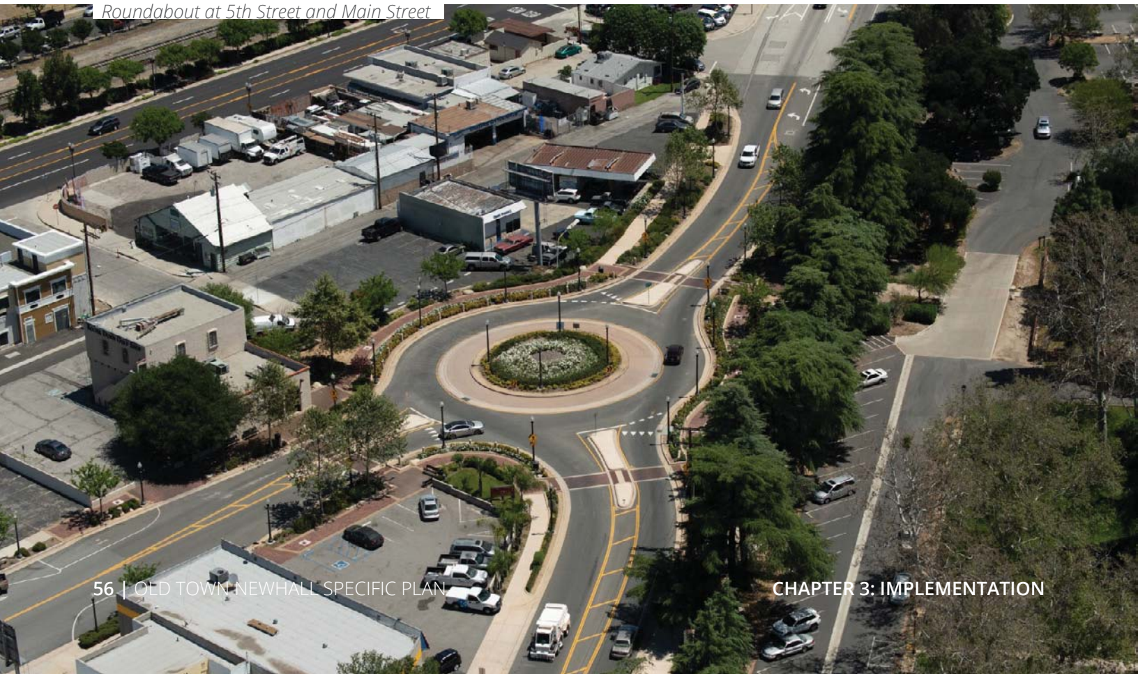
Roundabout at 5th Street and Main Street
