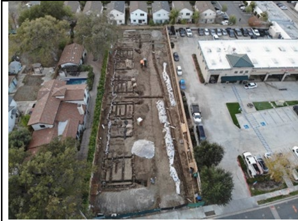
Existing: Looking West
