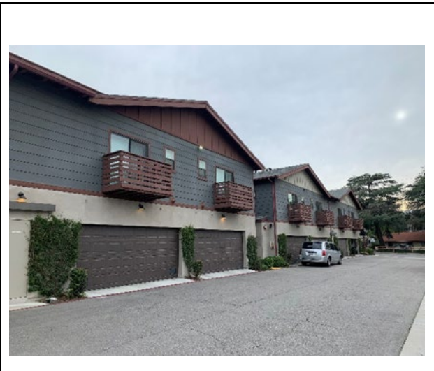
Existing: Looking Southwest
