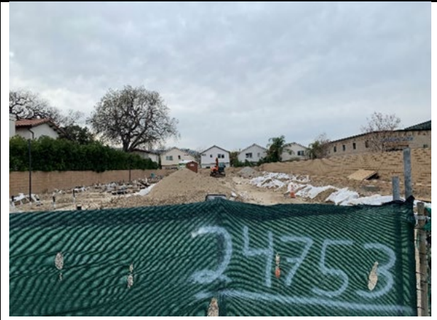
Existing: Looking West
