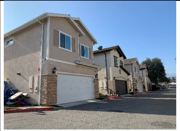
Existing: Looking Southwest
