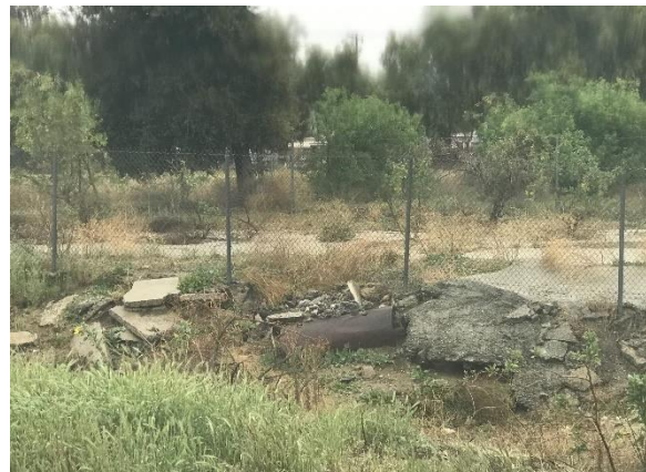
Abandoned Water Heater Shell Serving as Part of Rip-Rap Bordering Metropolitan Water District R-O-W (Which Tracks Eastern Boundary of Target Property). Drainage is Along Eastern Border and Flows North to join Placerita Creek .
