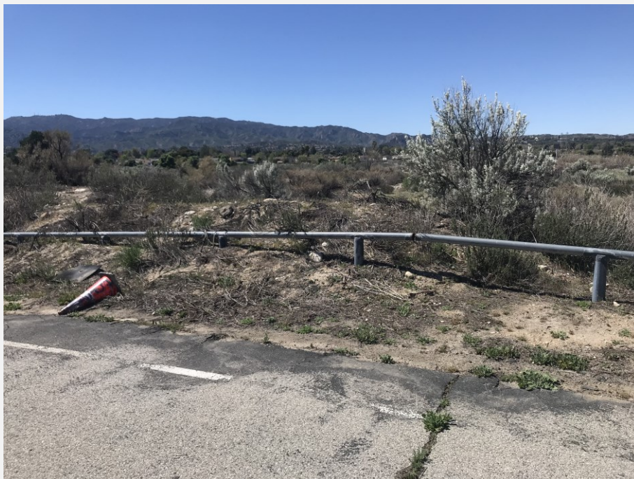
Photograph 26. View looking west from the Placerita Creek streambed east of the Project site's eastern boundary. (12)
