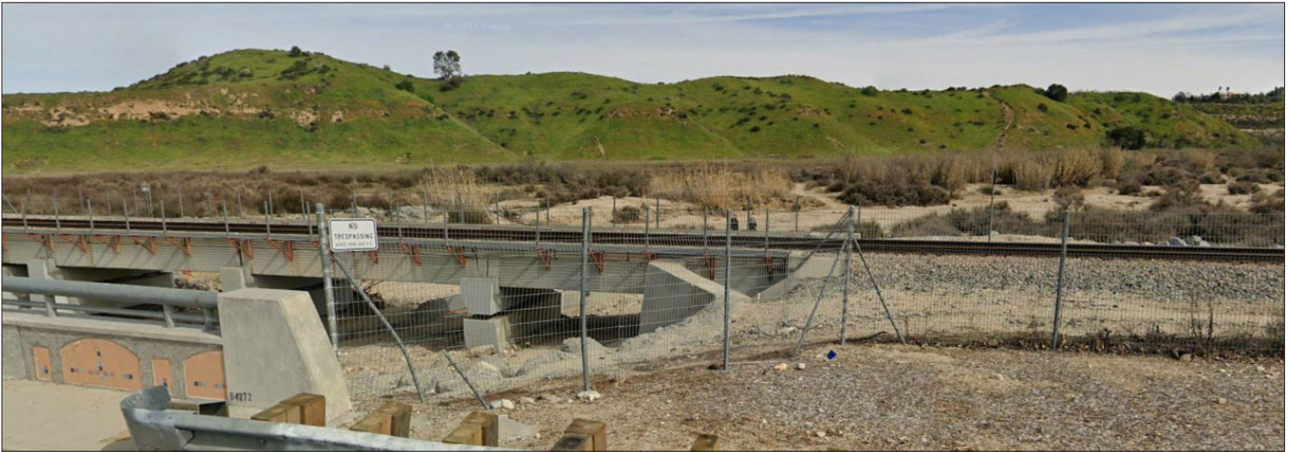
IMAGE 3: View into the northern portion of the Project Site facing northeast from Railroad Avenue and Placerita Creek. View shows the foreground views of Placerita Creek, the existing adjacent railroad right-of-way and associated culvert structure, and the ridgeline along the northern boundary of the Project Site.
