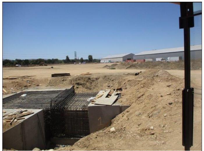
12. Storm drainage construction
