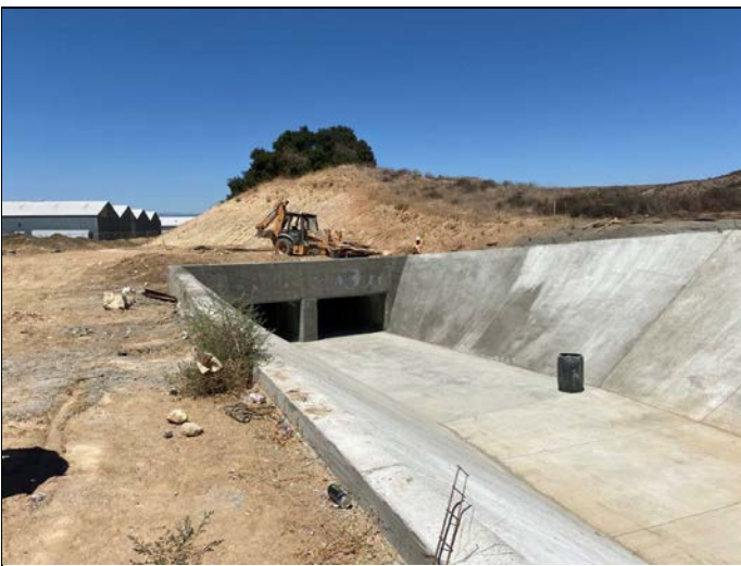
11. Storm drainage construction
