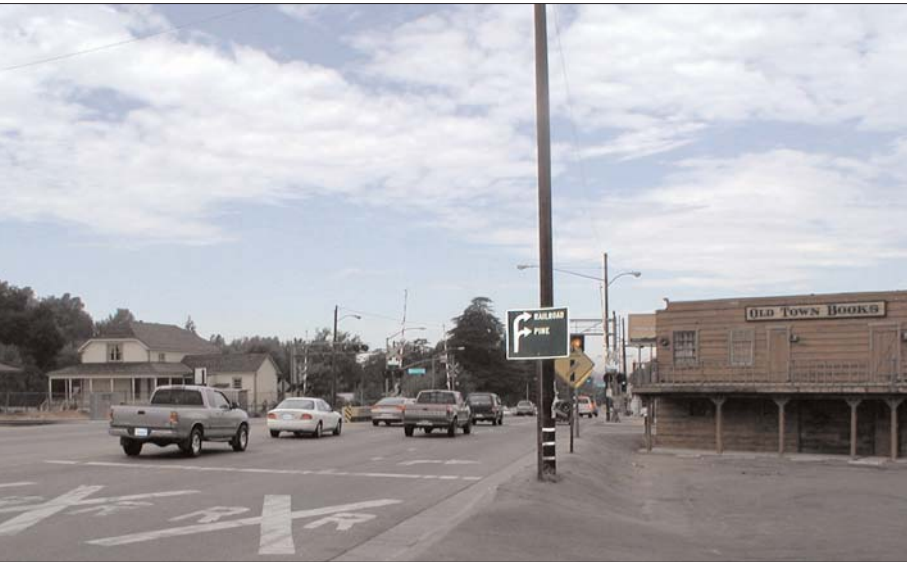
Overhead utilities at south entry to Downtown Newhall
