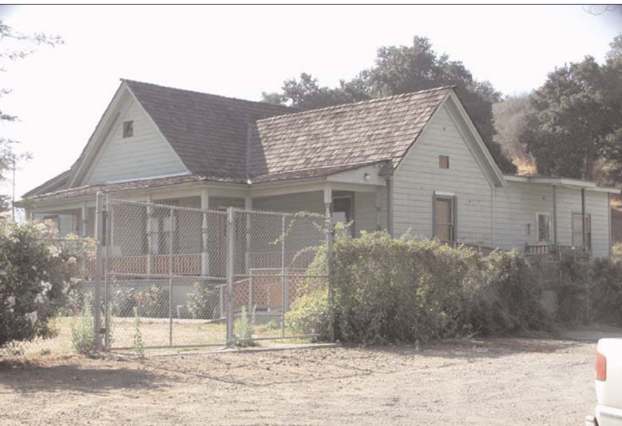
A. Visitorís Center: Historic Pardee House to be relocated at south entry to Downtown Newhall
