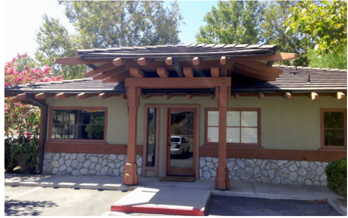
Example of commercial pad on Soledad Canyon Road and Lost Canyon Road
