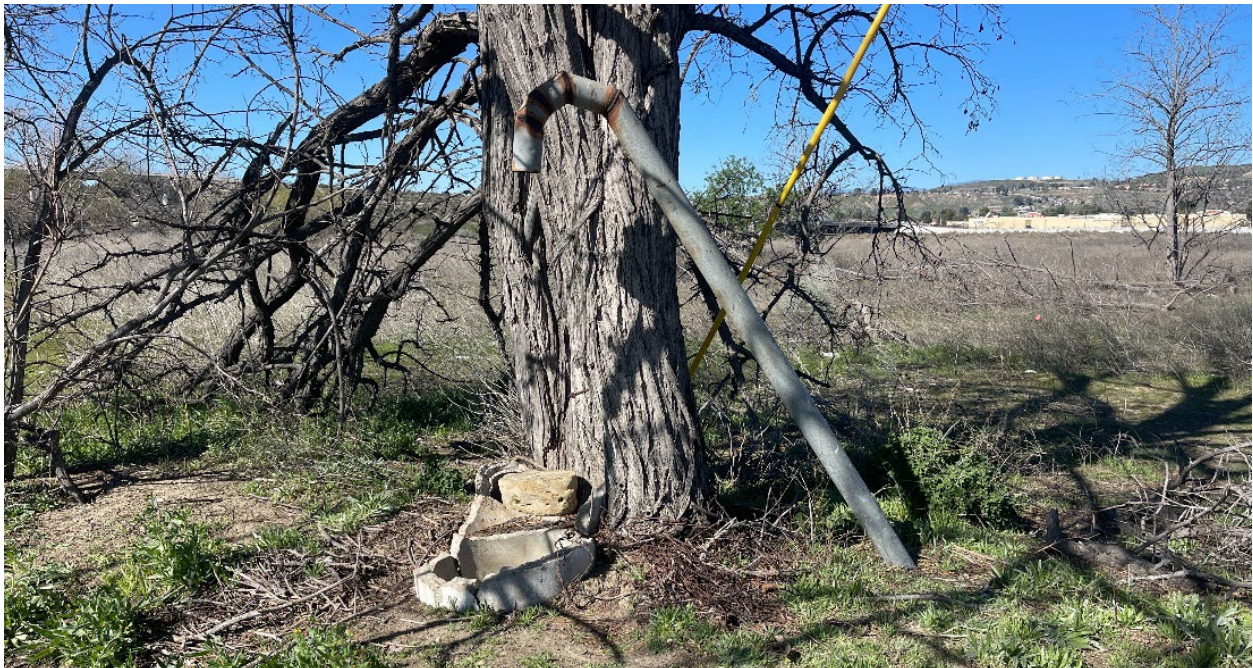
Photo 4. MBI-VP-01H Feature 4 - Metal water conveyance pipe and concrete cistern.
