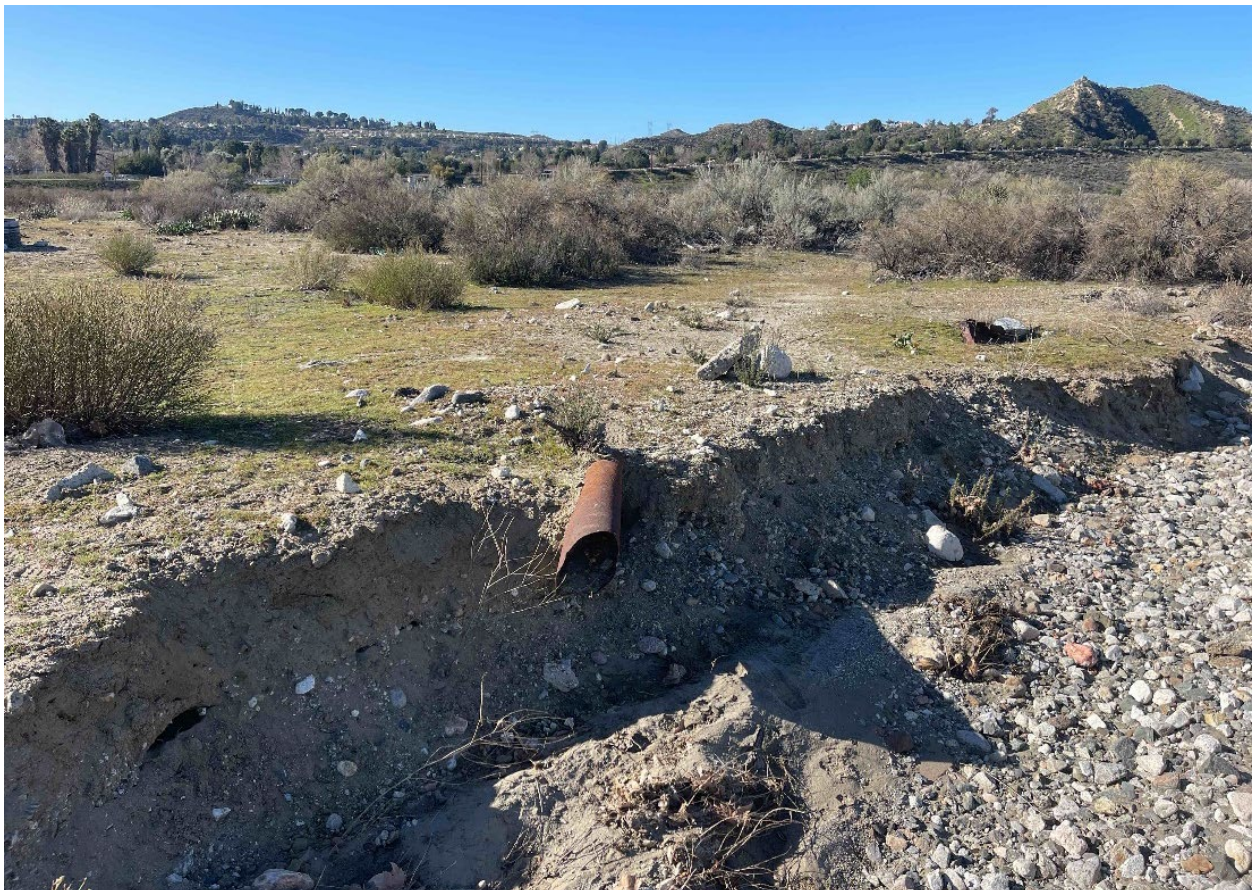
Photo 1. MBI-VP-MY-01H Feature 1 - Metal pipe jutting out into the Santa Clara Riverbed at the north end of the APE.
