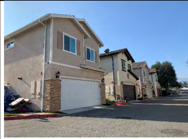
Existing: Looking Southwest
