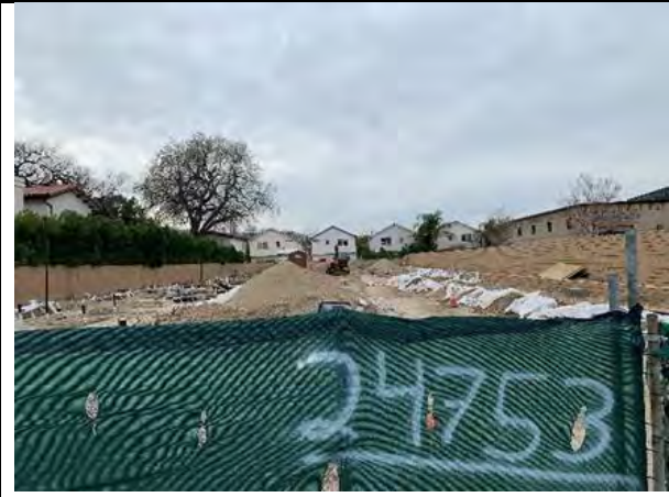
Existing: Looking West
