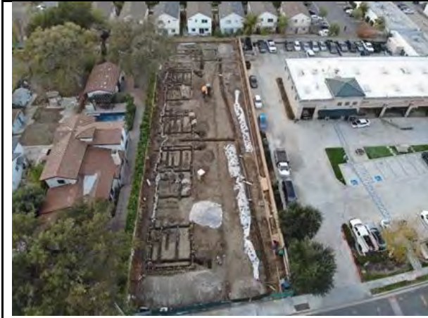
Existing: Looking West
