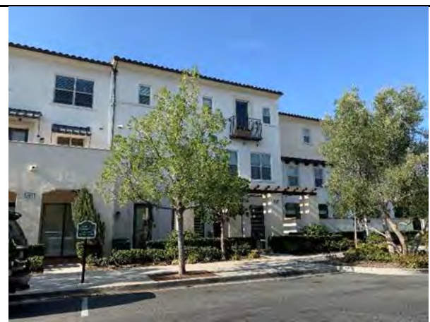
Existing: Looking West
