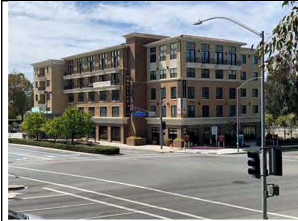
Existing: Looking Northwest
