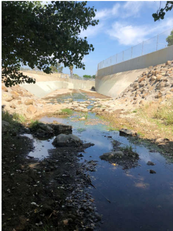
Photo 8 – Test Pit 1 facing north where IS-1 turns into concrete lined channel (6/3/20).
