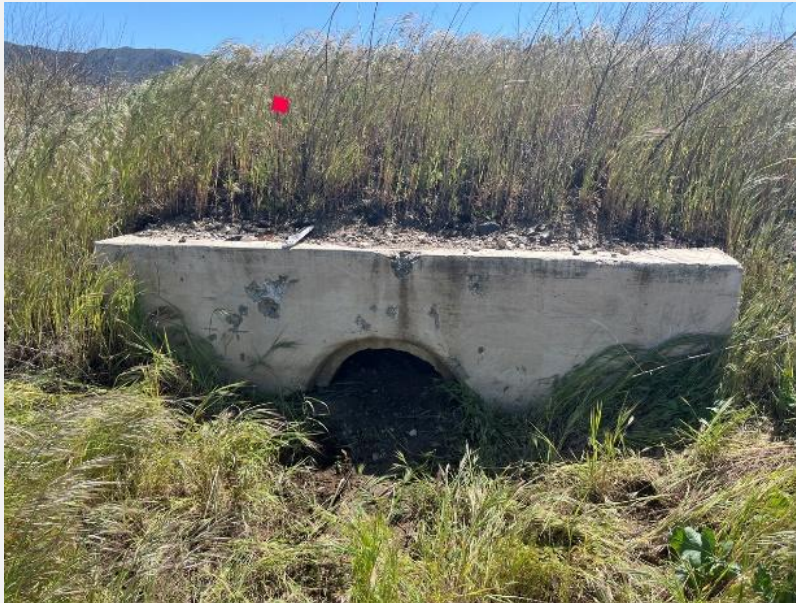
Exhibit 9. BSC-RB-S-001, Feature 3, concrete water conveyance system, view to the south.
