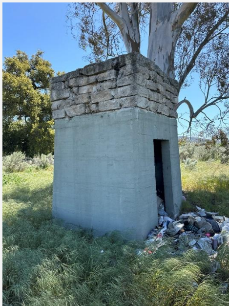
Exhibit 6. BSC-DF-S-006, Feature 4, standing structure, view to the southeast.
