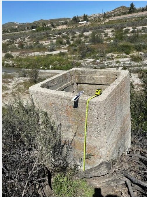
Exhibit 5. BSC-DF-S-005, concrete cistern, view to the northwest.
