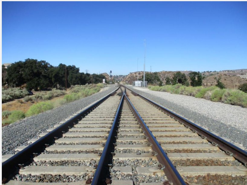
Exhibit 11. View of the SPRR Soledad Canyon Line segment, view looking west. 9/25/2025.
