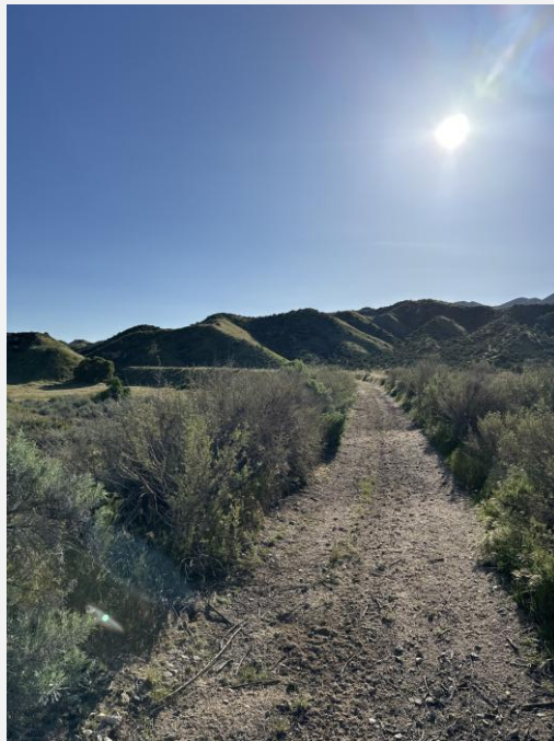
Exhibit 7. BSC-RB-S-001, Feature 1, earthen embankment, view to the east.
