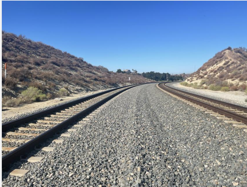
Exhibit 12. View of the SPRR Soledad Canyon Line segment, view looking west. 9/25/2025.
