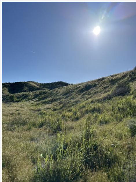
Exhibit 8. BSC-RB-S-001, Feature 1, earthen embankment, view to the southeast.
