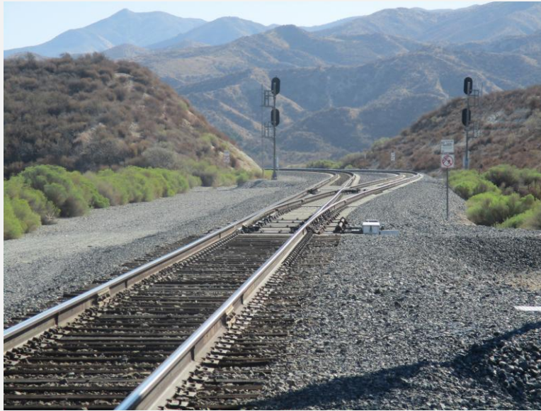
Exhibit 10. View of the SPRR Soledad Canyon Line segment, view looking northeast. 9/25/2025.
