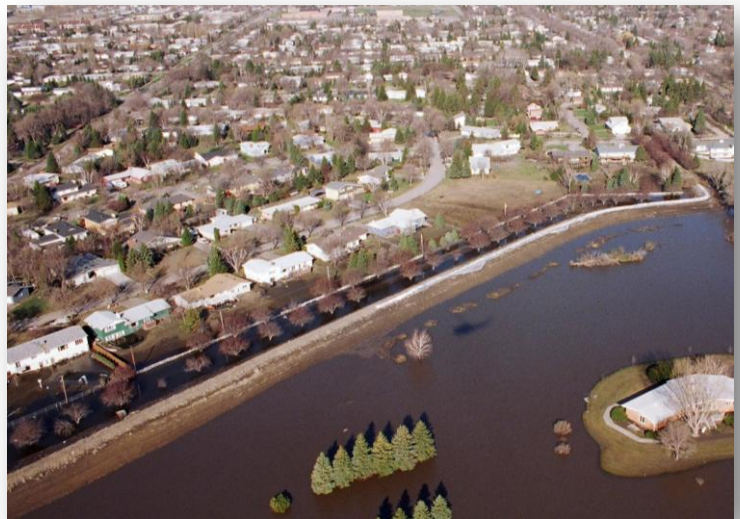
Accredited levees may help prevent properties from being flooded during the 1-percent-annual-chance flood.
